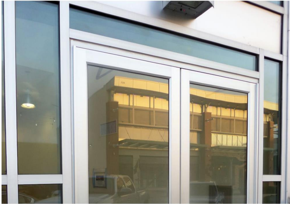
4 | NEW ANODIZED ALUMINUM STOREFRONT
